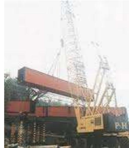
If the construction bridge is less 15 m long, there will need only one crane with maybe 21ton ability.
