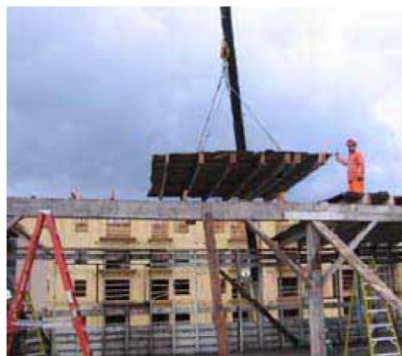
Fig. 13 panelization of roof structure
