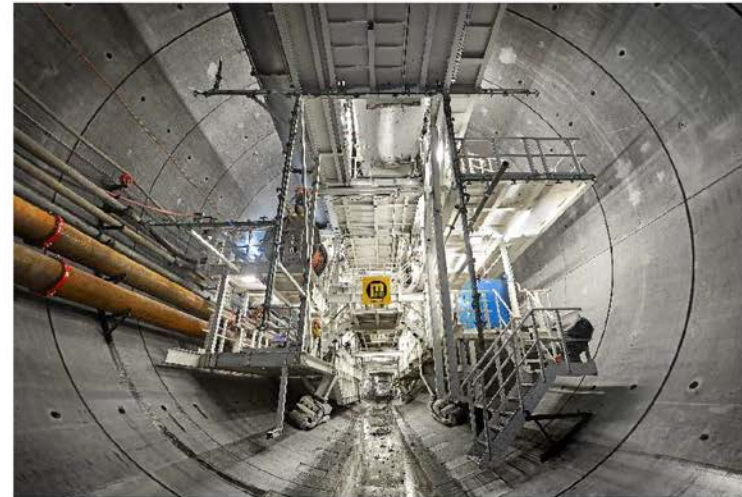
Mechanized tunneling, source: ILF
