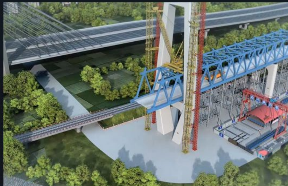
Steel beam hoisting simulation of yancheng bridge
