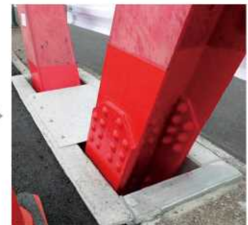
After repair (installation opening)
