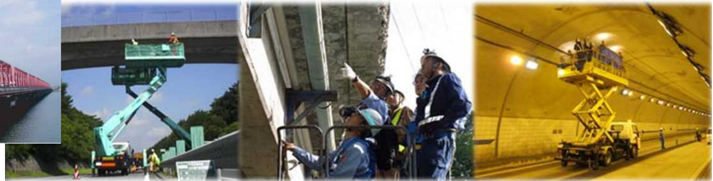
Close-range visual inspection
